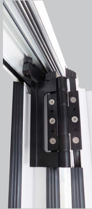
View of upper retained roller hinge
