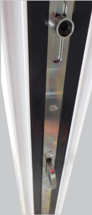
View of lower hook bolt and cam
